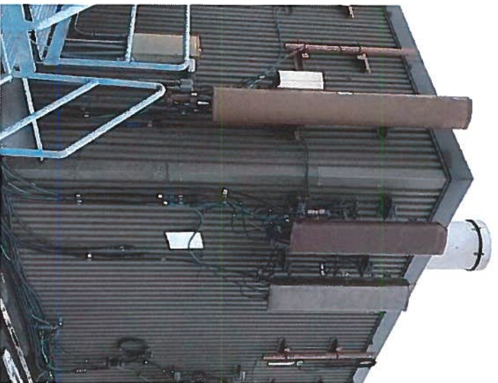
Gamma Sector Pipe Mounts (Typ.)
